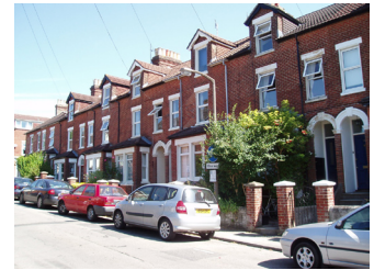
Queen's Road - brick elevations, tiled roofs, chimneys, bays, low boundary walls
