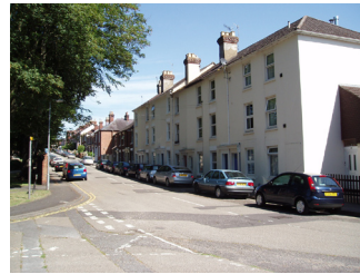
College Street Junction - render, hipped roof, chimneys, back-of-footway
