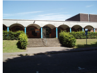
Swimming Pool Building - front
