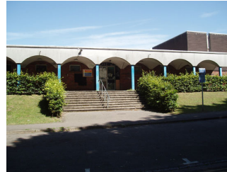
Swimming Pool Building - front
